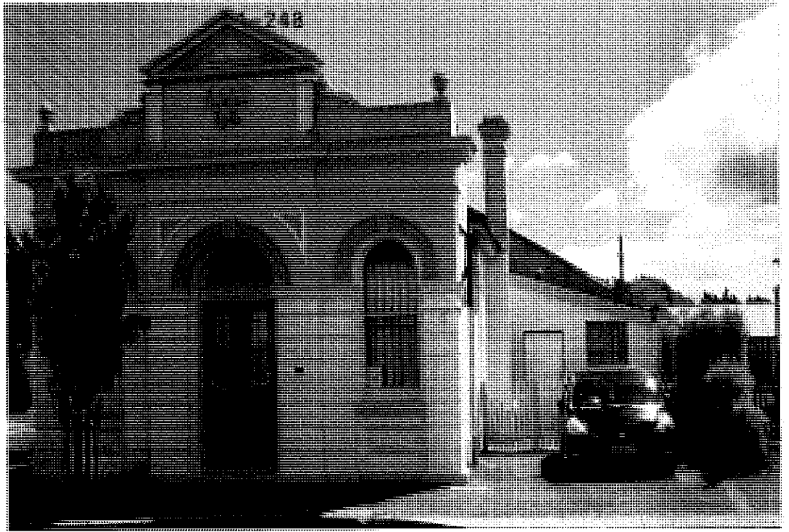
PHOTO TAKEN MARLBOROUGH ST. - FRONT VIEW OF BUILDING
