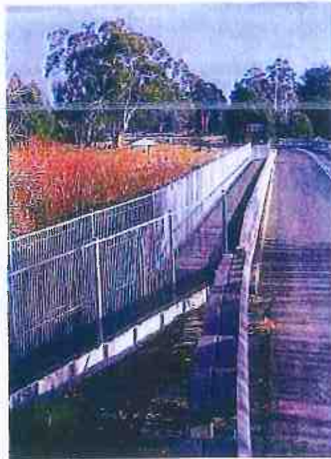
Existing pedestrian access way over river
