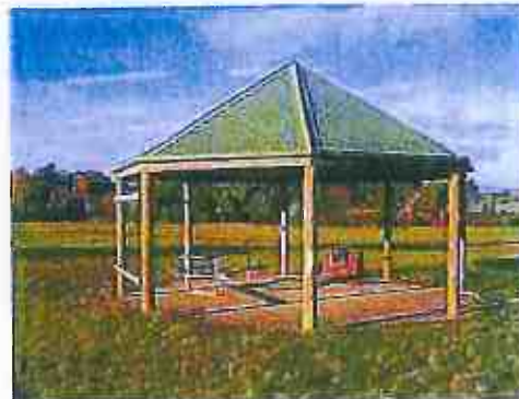
Existing gazebo structure
