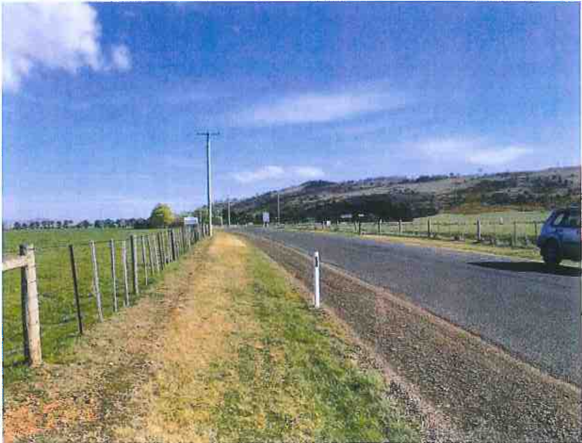
Photograph 1 - View to left, back to Midland Highway
