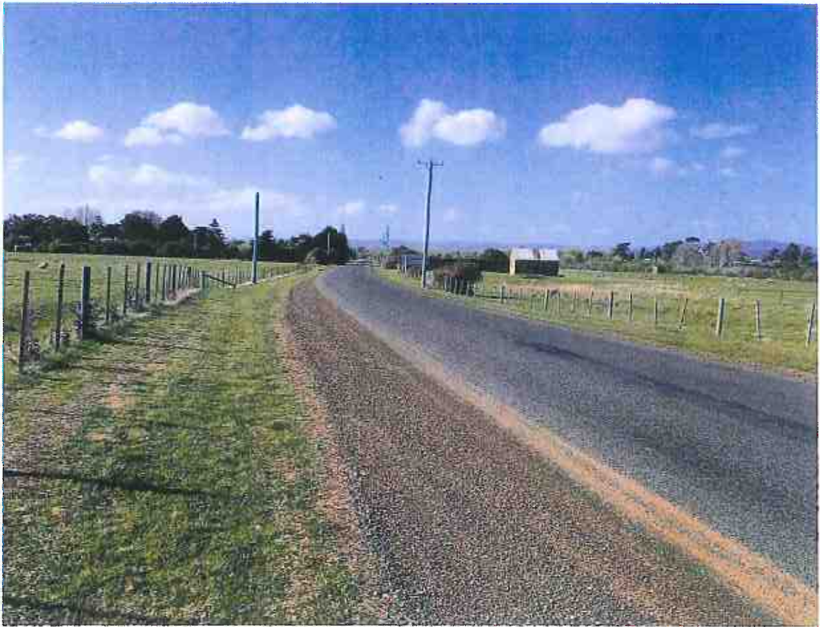
Photograph 3 - Typical Roseneath Road Profile
