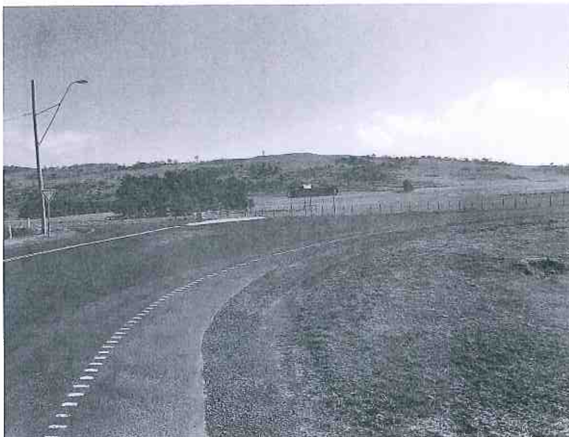
Photograph 4 - Intersection at Midland Highway
