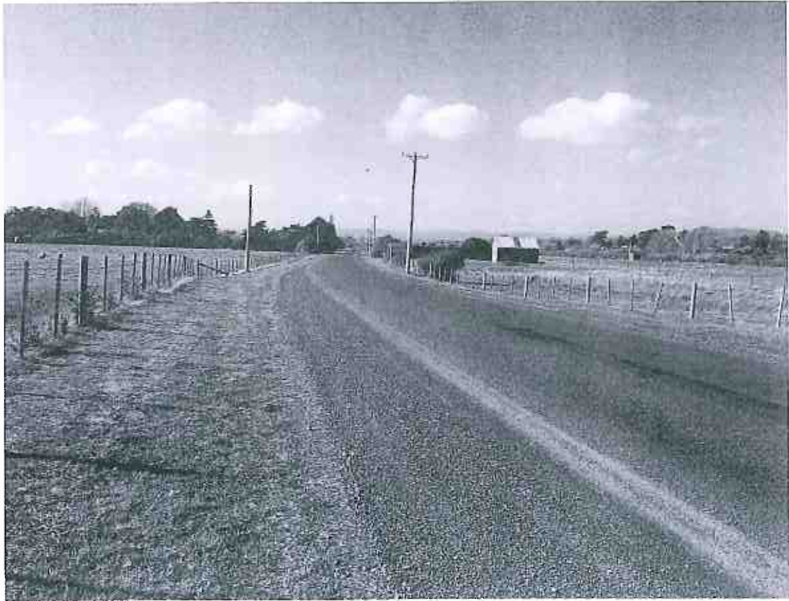
Photograph 3 - Typical Roseneath Road Profile
