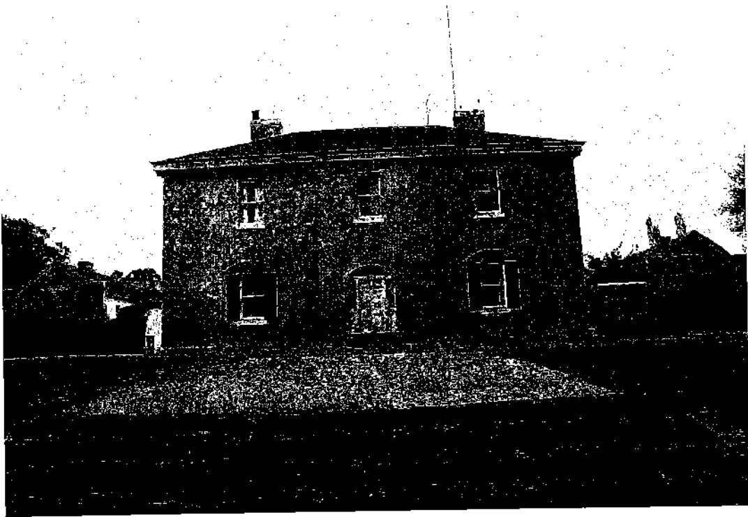
Figure 2.4 – The façade (northern elevation) of the Symmons Plains homestead, the outbuildings can be seen on each side.
