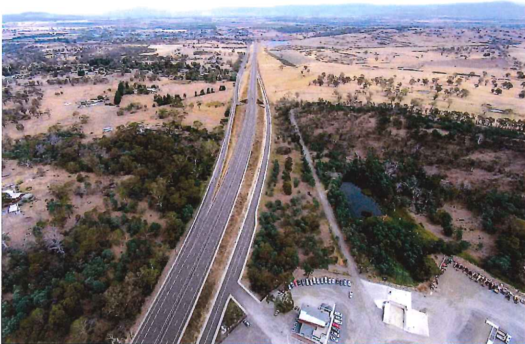
FIGURE 4 LOOKING SOUTH TOWARDS PROPOSED UNDERPASS
