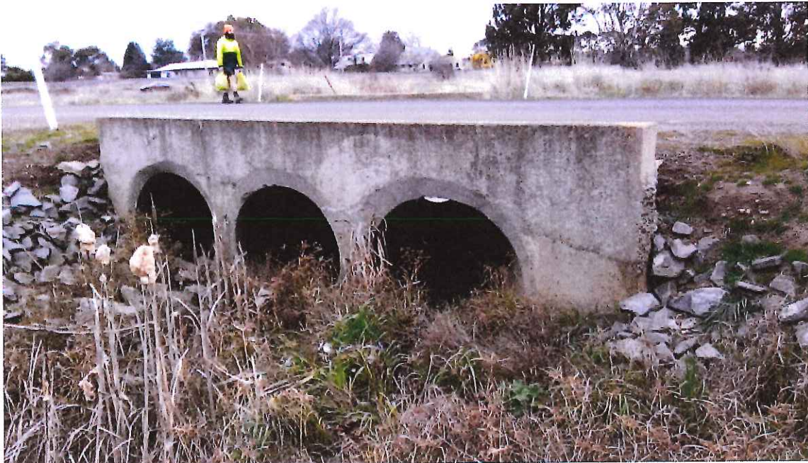
Figure 3. Edward Street culverts (upstream/inlets)
