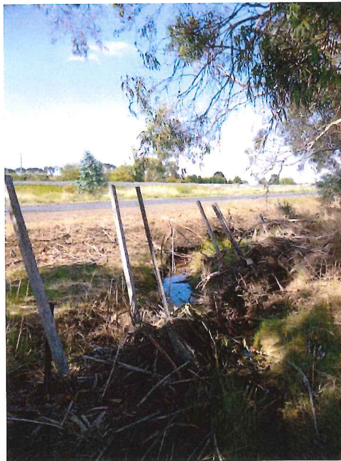
Figure 8. Existing channel view south from approximate chainage 160m
