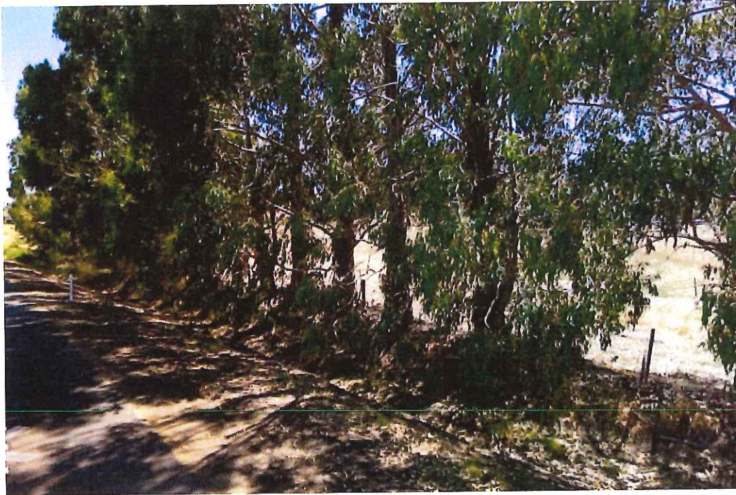
Figure 9. Existing swale view southwest from approximate chainage 120m
