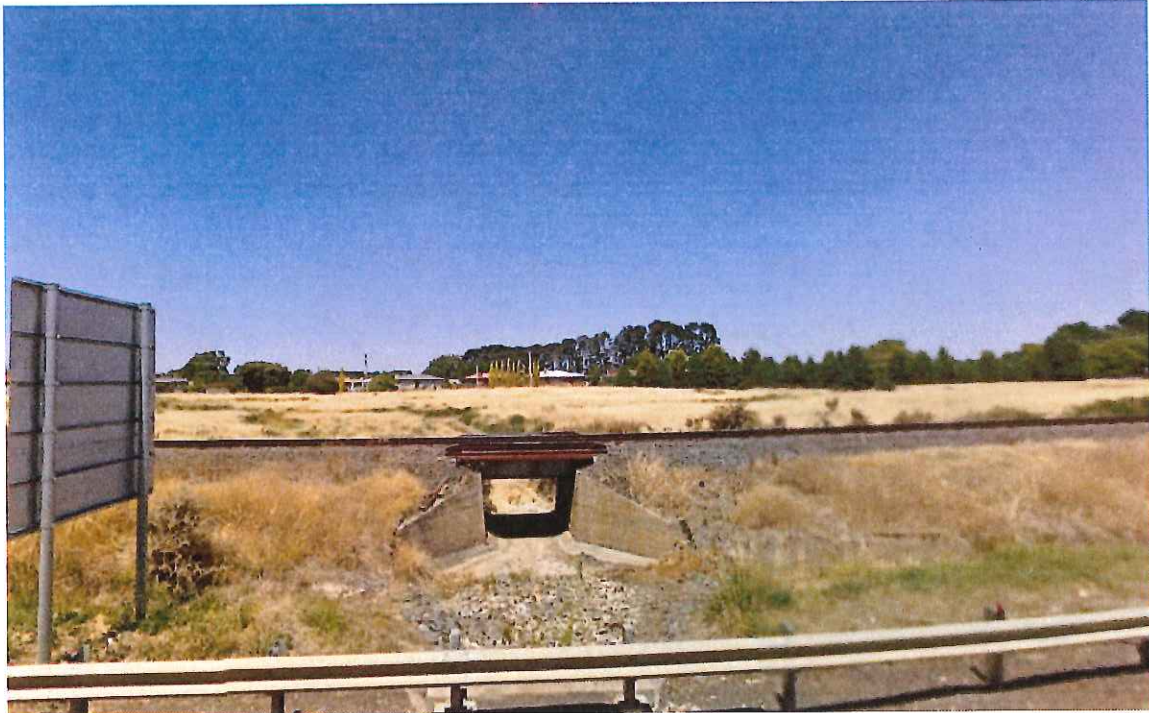
Figure 12. Rail bridge view east from Youl Road
