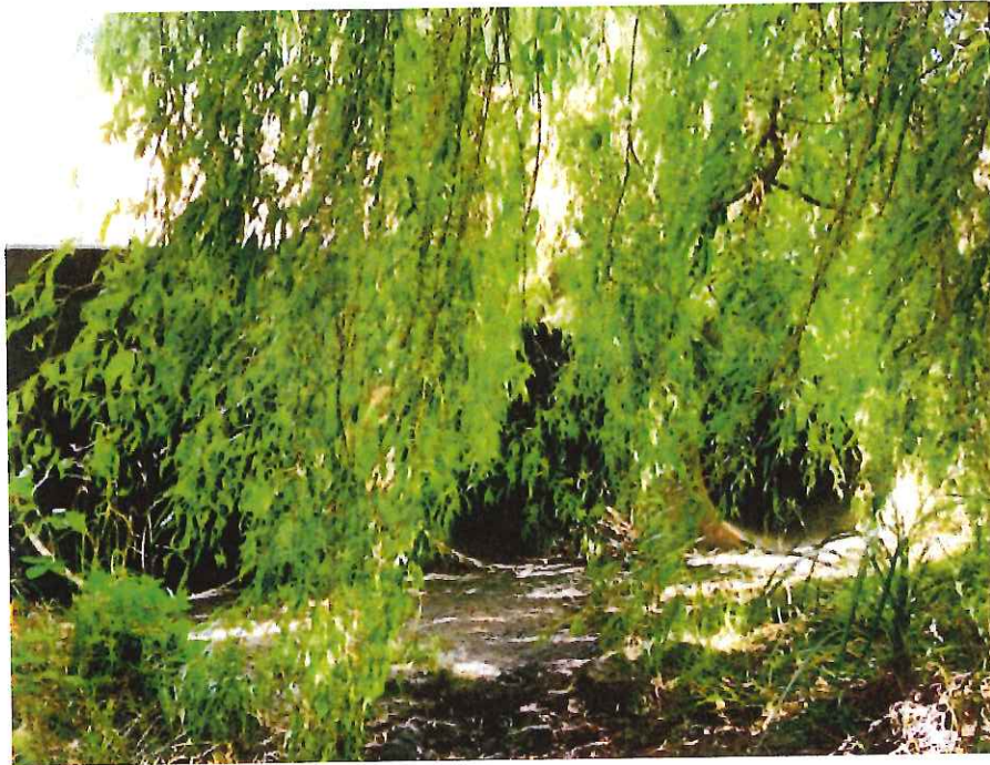
Figure 16. View of creek widening upstream to Old Cemetery Road
