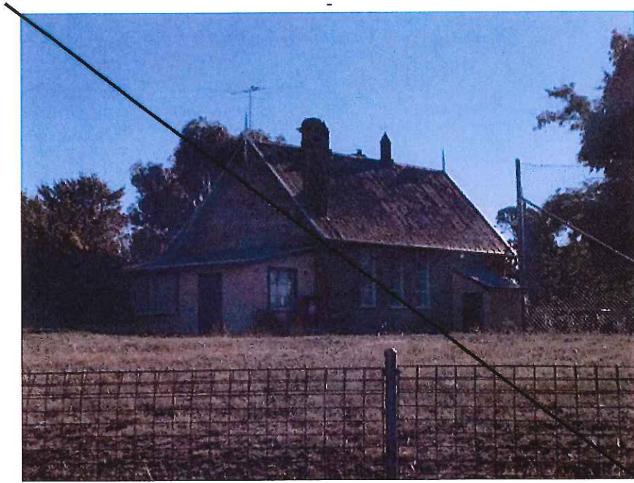
Figure 9 — 14 to 18 Bridge Street, old School building
