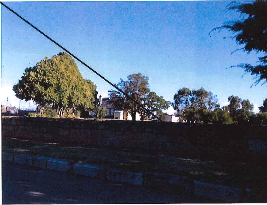
Figure 7 – 14 to 18 Bridge Street, view from Bridge Street
