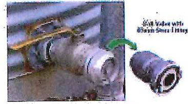
Figure 9 - STORZ 65mm
