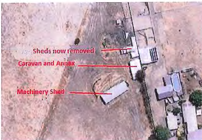
Figure 2 – Uses in the immediate area
