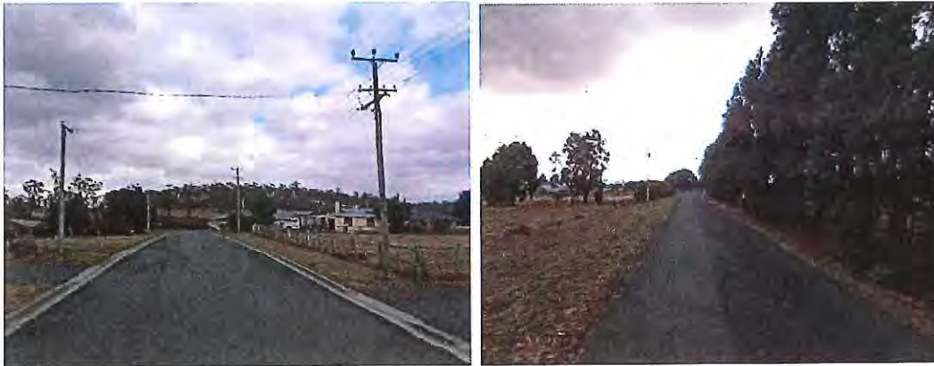
Figure 5 and 6 – Access Road – Fully formed section and part formed section
