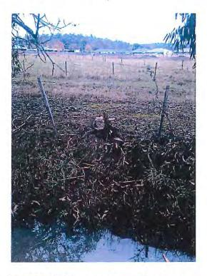
Figure 5. – Stump of tree that fell into road reserve late last year. Notice location of tree in relation to open drain and the exposed root structure.
