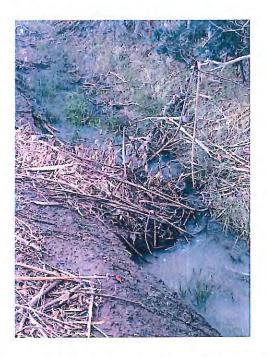
Figure 3. – Debris from shedding Eucalypts in the open drain.
