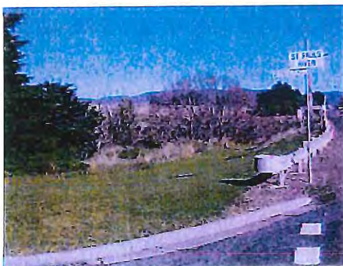
The existing easement near Boucher Park
