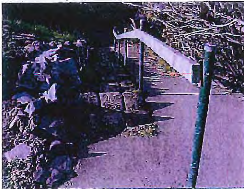
Existing stairs/ramp near railway underpass
