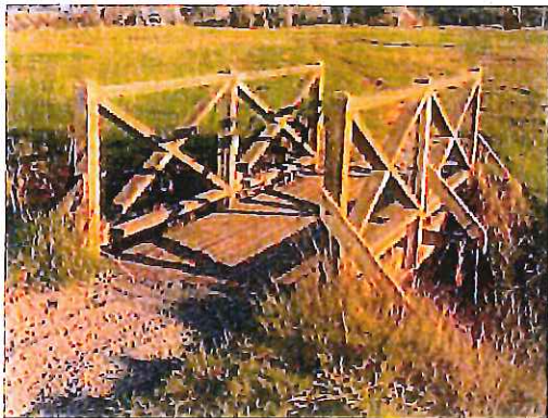
Existing footbridge over drainage channel
