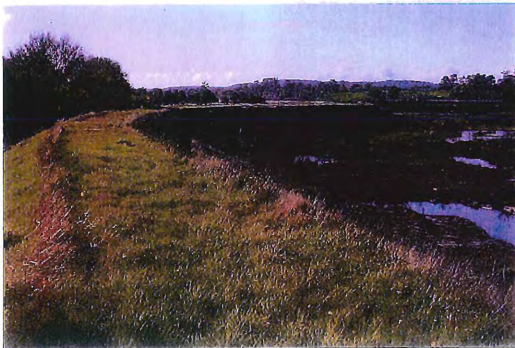
The existing levy bank tops provide level, elevated, well-drained, flood free platforms for trail development
