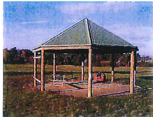
Existing gazebo structure
