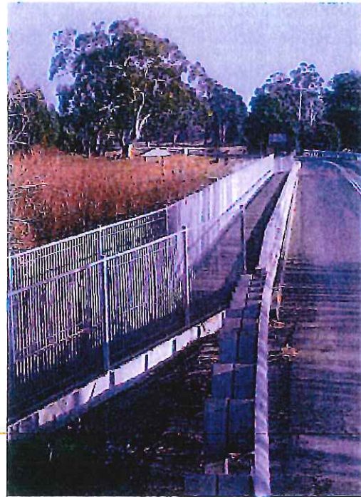
Existing pedestrian access way over river
