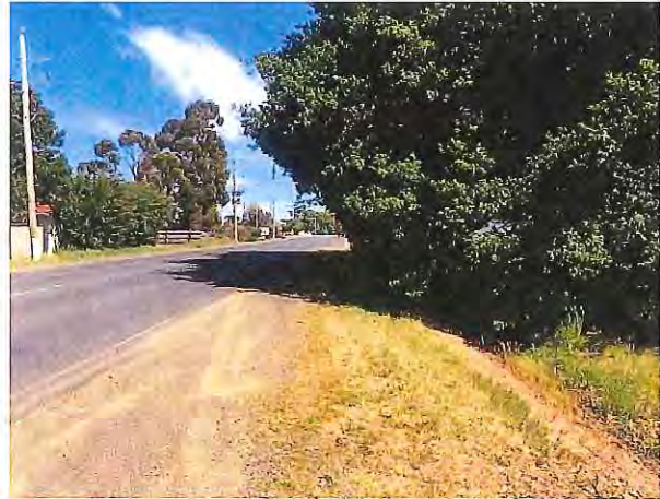
Figure 5: Sight Distance to South (northbound vehicles)
