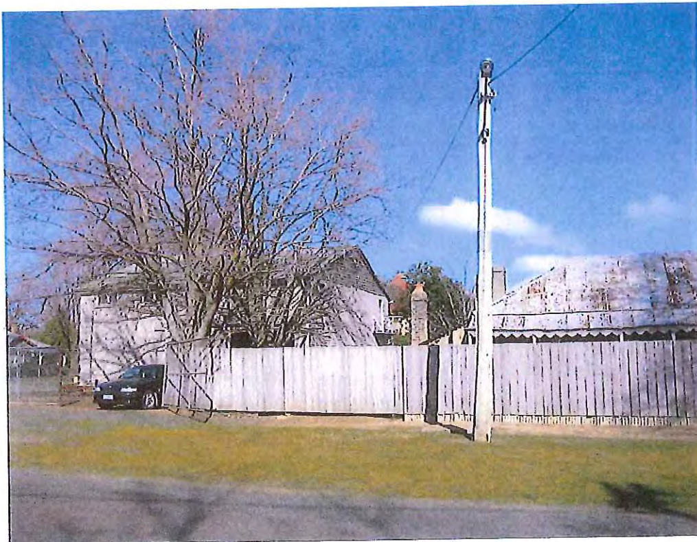
North & West Wall From High Street.
