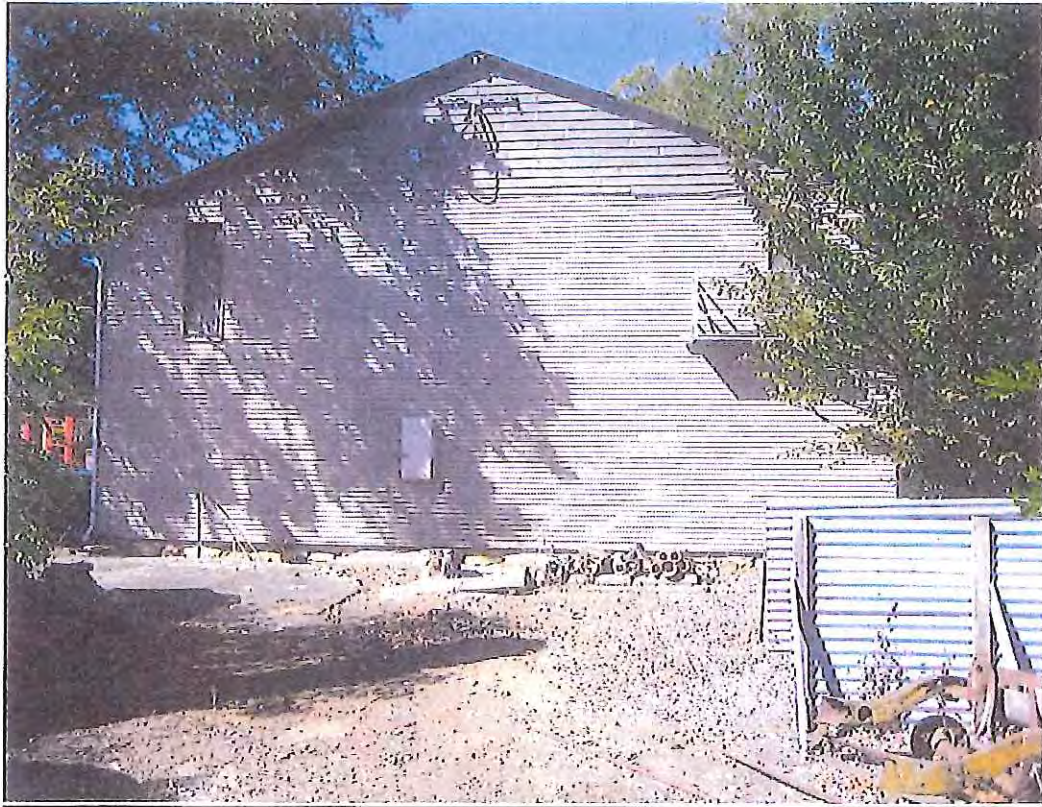
West Wall ( Rear of Building )
