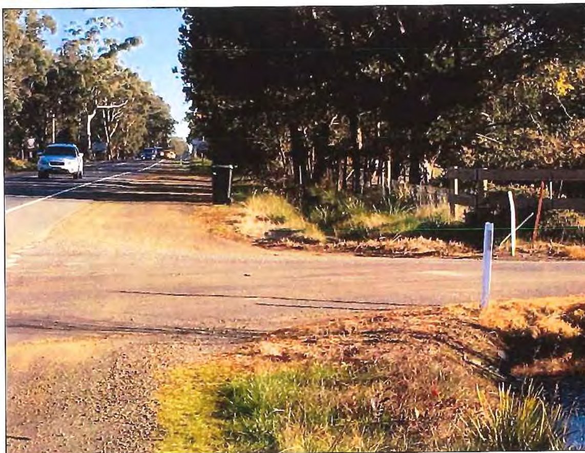
FIGURE 4: SOUTHERN END LOOKING NORTH FROM BELLEVUE RD
