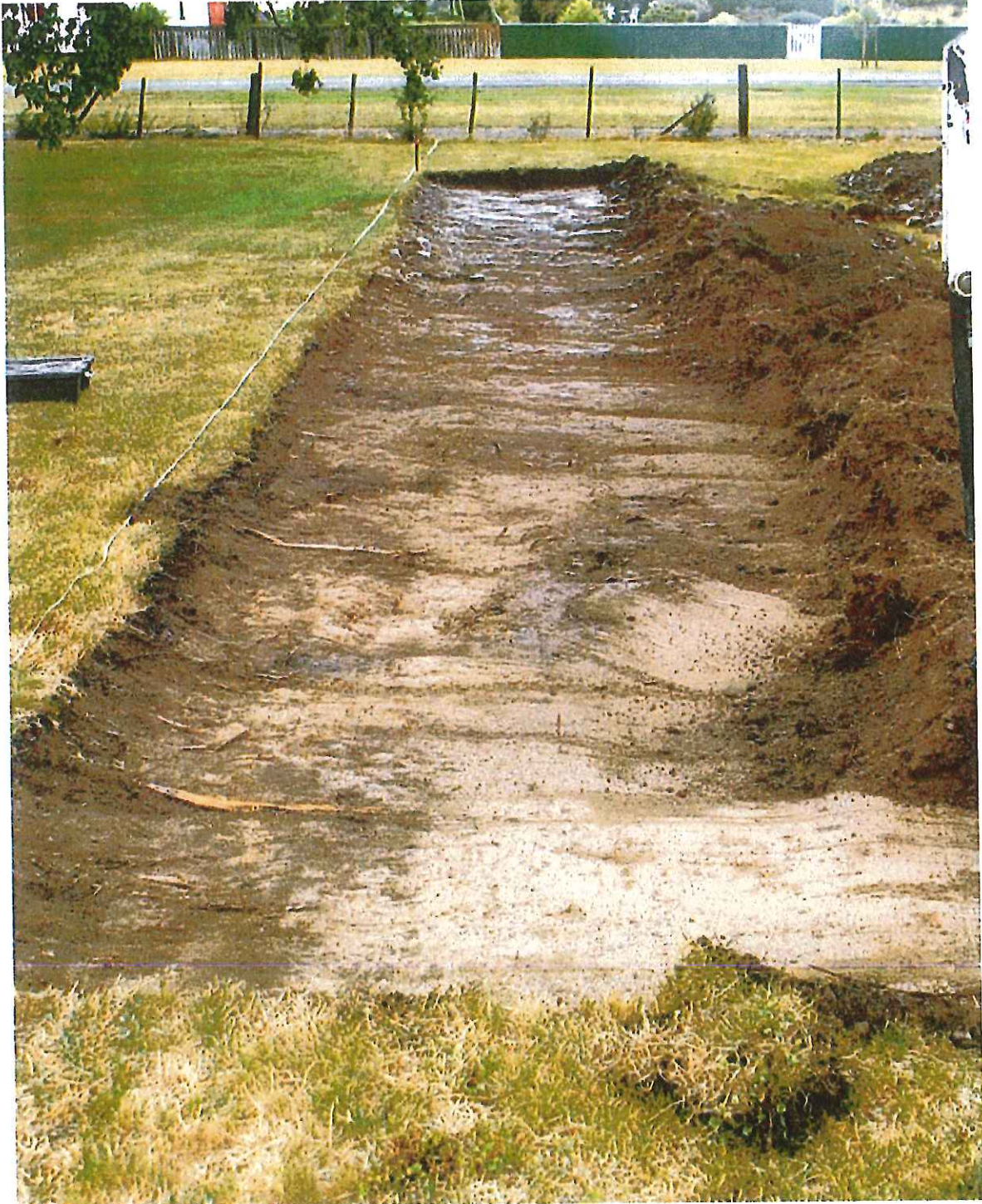
Figure 3.2 – The northernmost portion of the excavation area following removal of topsoil.
