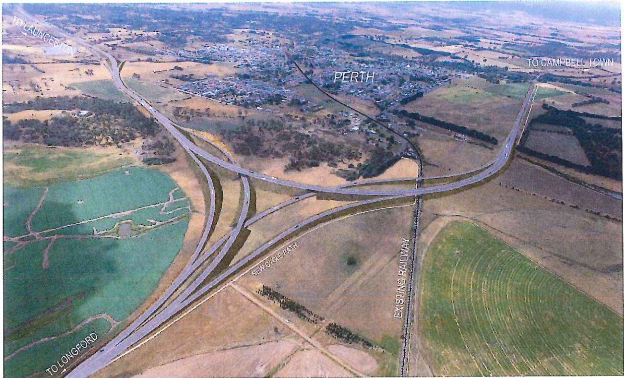
FIGURE 9-3 WEST OF PERTH LOOKING EAST
