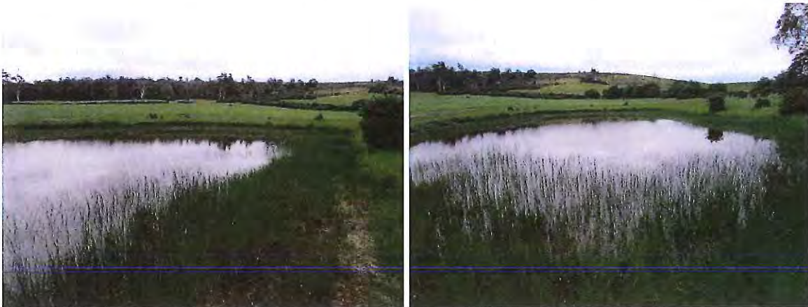
Views of Sheepwash Corner dam (20 Nov. 2014) – note the substantial change in condition between 2014 and 2017
