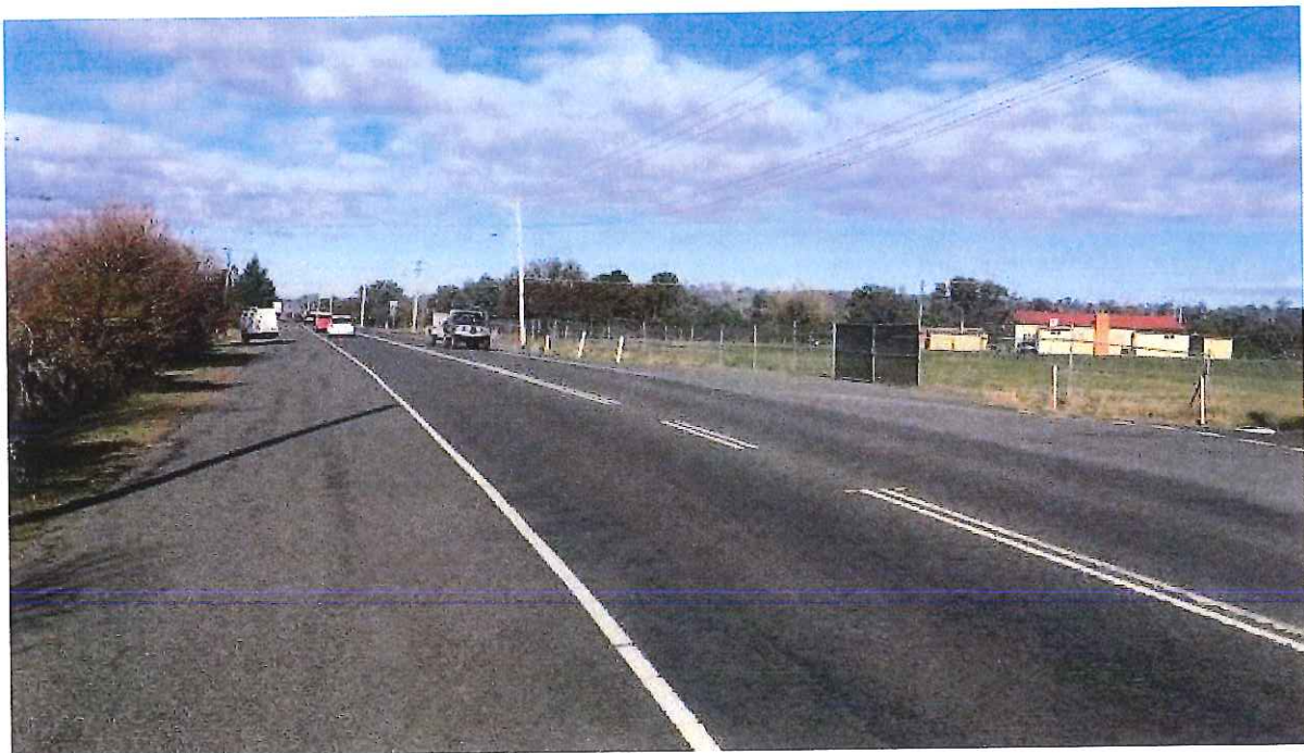
Figure 2.3: View of the site along High Street from the north
