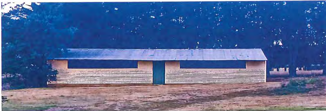
Figure 15 – Existing storage shed.
