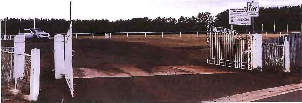
Figure 8 – Macquarie Street main entry.
