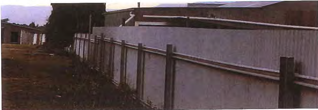
Figure 7 – Metal colorbond fence along the full length of the western boundary.
