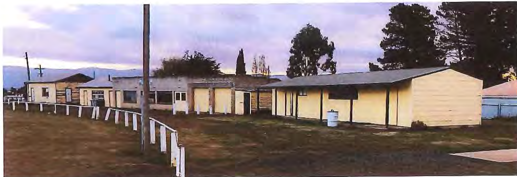
Figure 13 – Existing clubhouse and visitor change room building.
