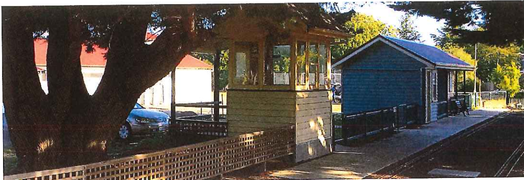
Figure 26 – Existing miniature railway station and control building.
