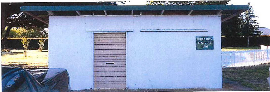
Figure 23 – Existing old change room.
