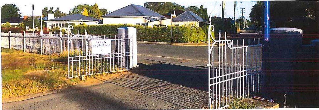
Figure 9 - Barclay Street main entry.
