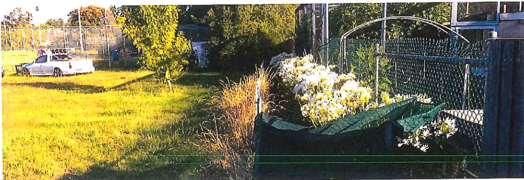
Figure 8 – South western boundary consists of a variety of residential fences.
