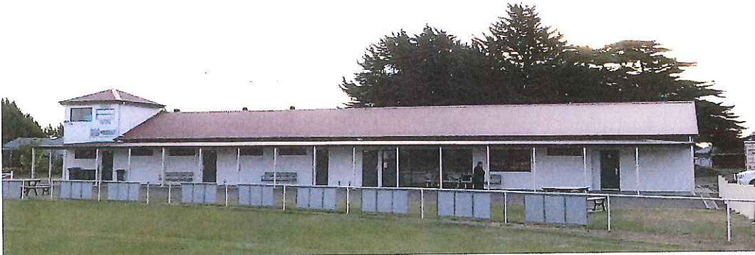
Figure 22 – Existing clubhouse and change rooms.
