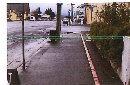
Image 13: Pavement lift along High Street
