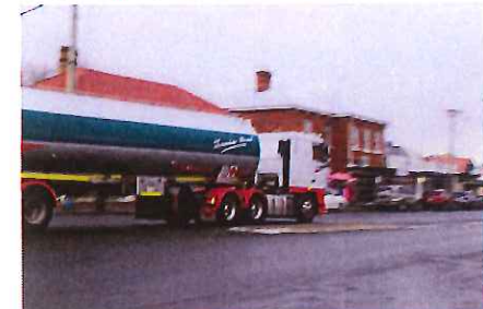
Image 12: Limitations due to road narrowing over Red Bridge
