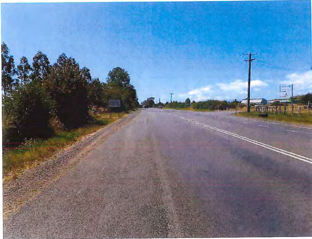
Photograph 4.1: View to north along Hobart Road with junction of McGraths Road on right
