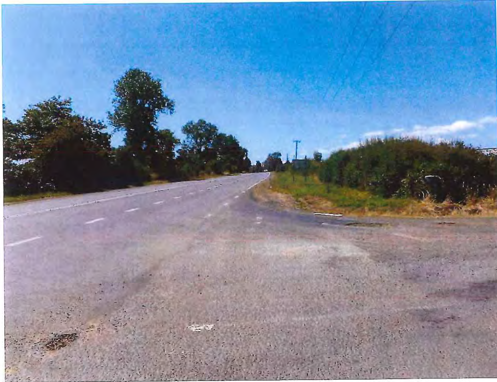
Photograph 6.2: View to north along Hobart Road from McGraths Road
