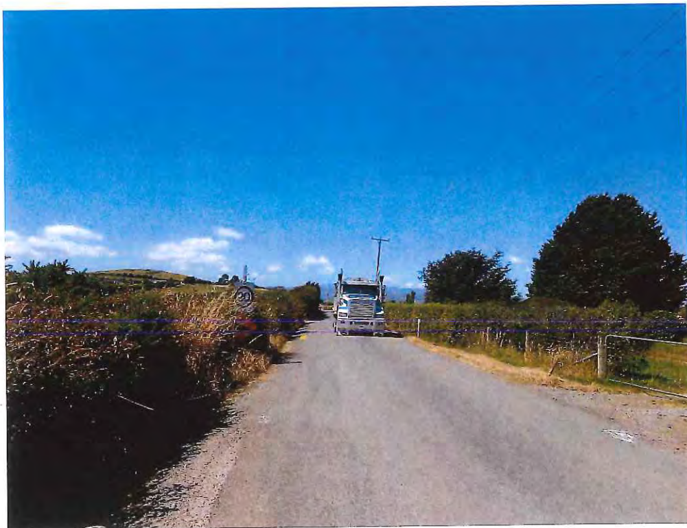
Photograph 4.4: View to east along McGrath Road around 260m east of Hobart Road
