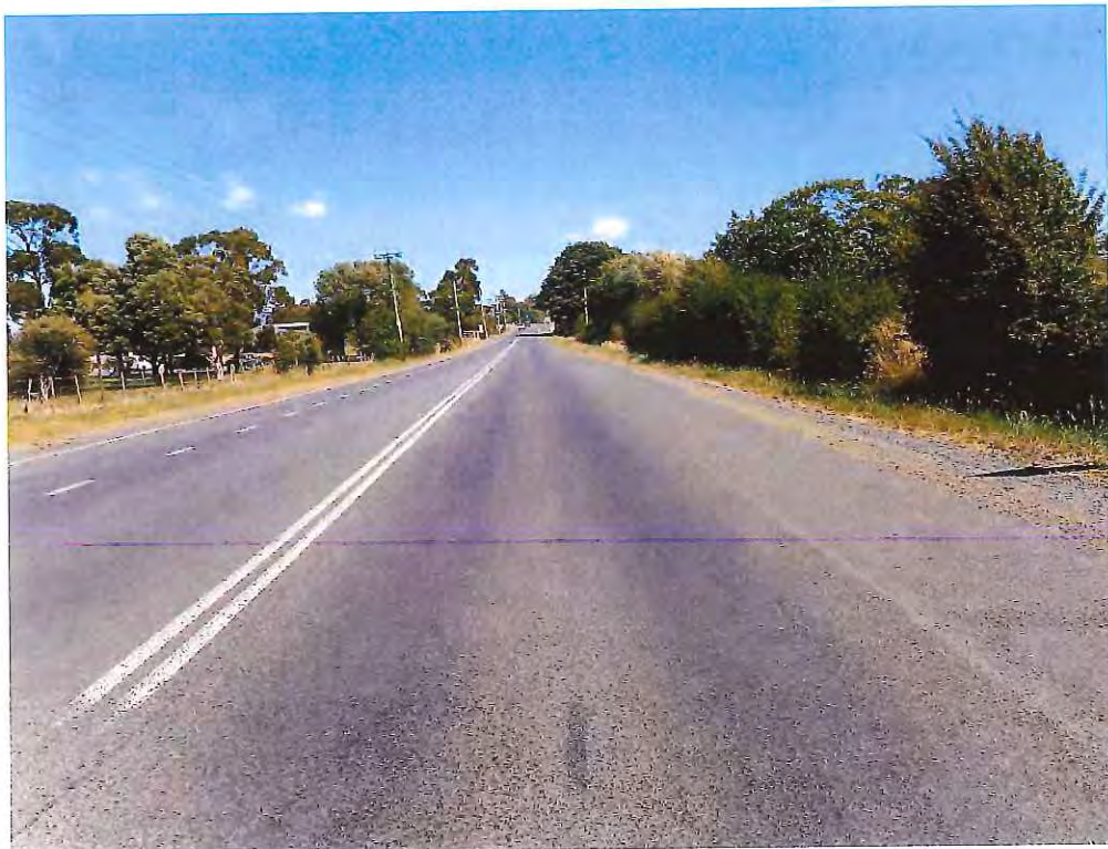
Photograph 6.5: View to south along Hobart Road from rear of vehicle turning right into McGraths Road
