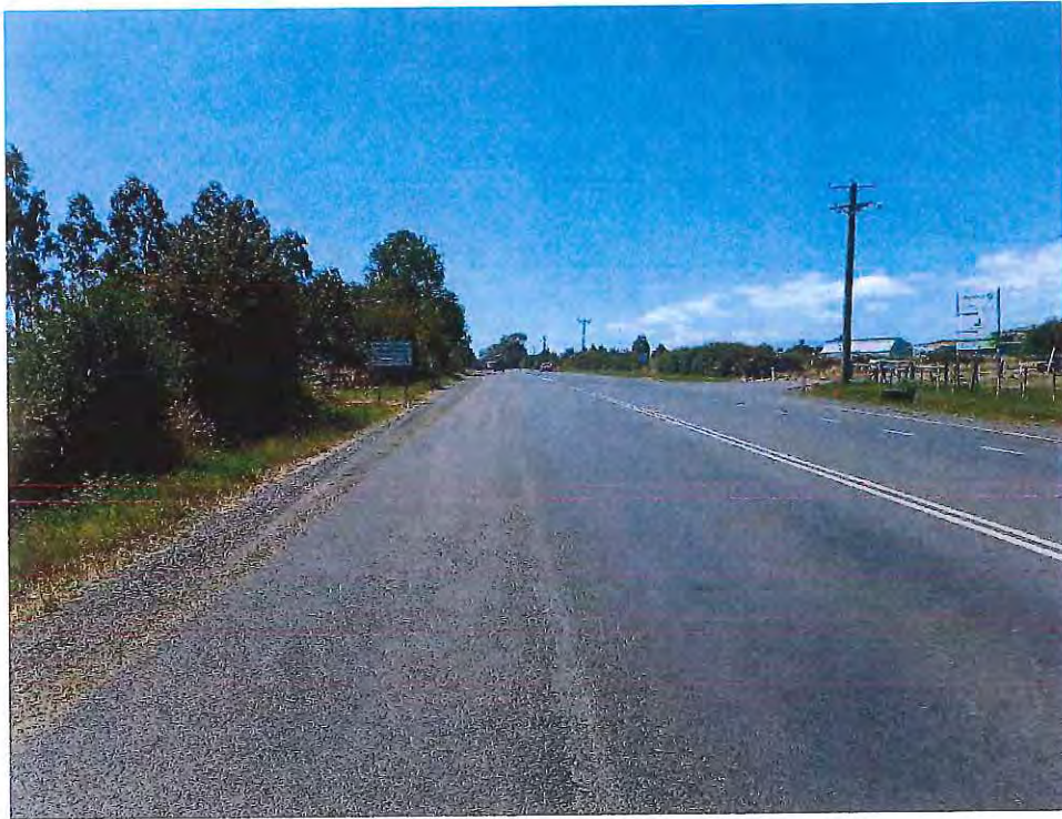
Photograph 4.1: View to north along Hobart Road with junction of McGraths Road on right
