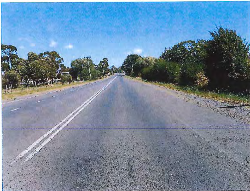
Photograph 6.5: View to south along Hobart Road from rear of vehicle turning right into McGraths Road
