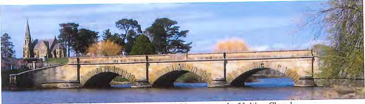
View of Council owned land beyond the Ross Bridge next to the Uniting Church
