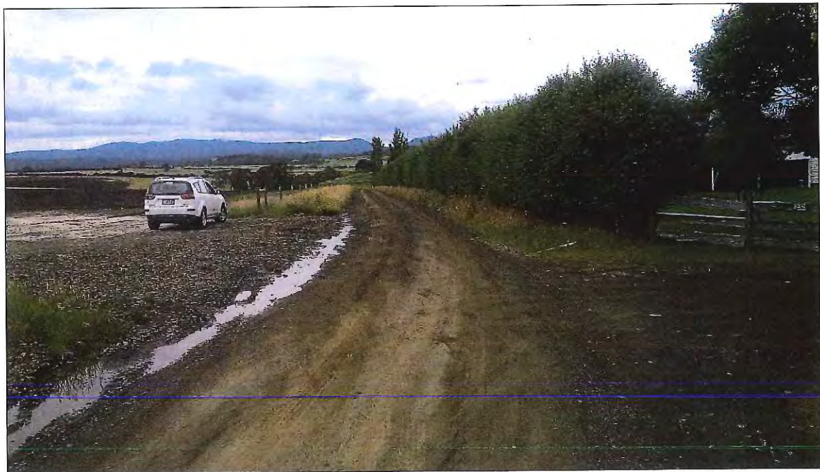
Image 4 - Looking northeast along Egerton Road. Vehicle is parked within proposed exit driveway. Available sight distance in excess of 190m.
