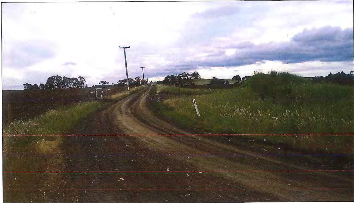
Image 3 - Looking northwest along Egerton Rod from the road corner. Available sight distance is in excess of 380m from site entrance on right hand side.
