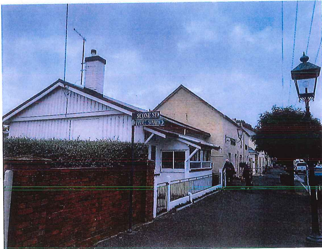
Image 4. Buildings at Numbers 6 and 8 Russell Street
