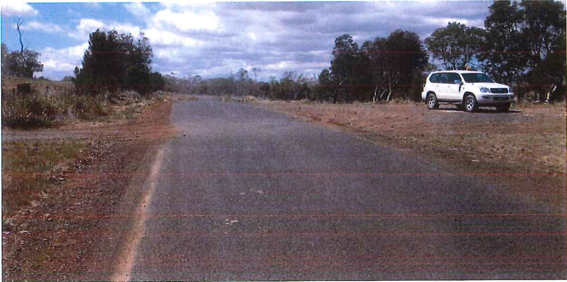
Pull-off Bay looking east, adjacent to the Quarry Entrance
