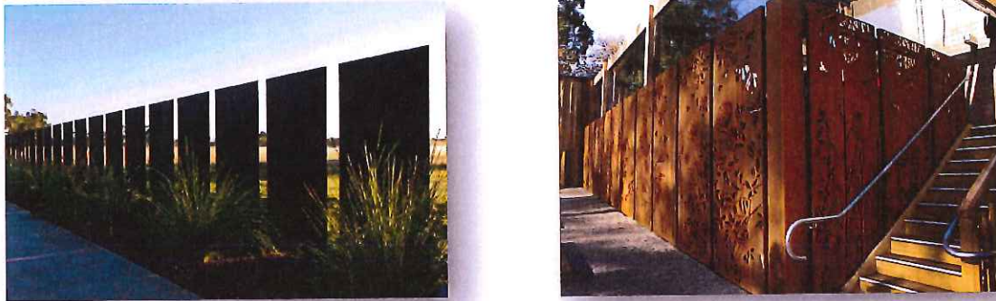
Figure 5 – Potential fencing options may include gaps, cut-outs or transparent infill to capitalise upon views whilst maintaining privacy.
