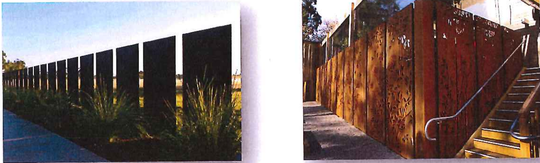
Figure 7 – Potential fencing options may include gaps, cut-outs or transparent infill to capitalise upon views whilst maintaining privacy.
