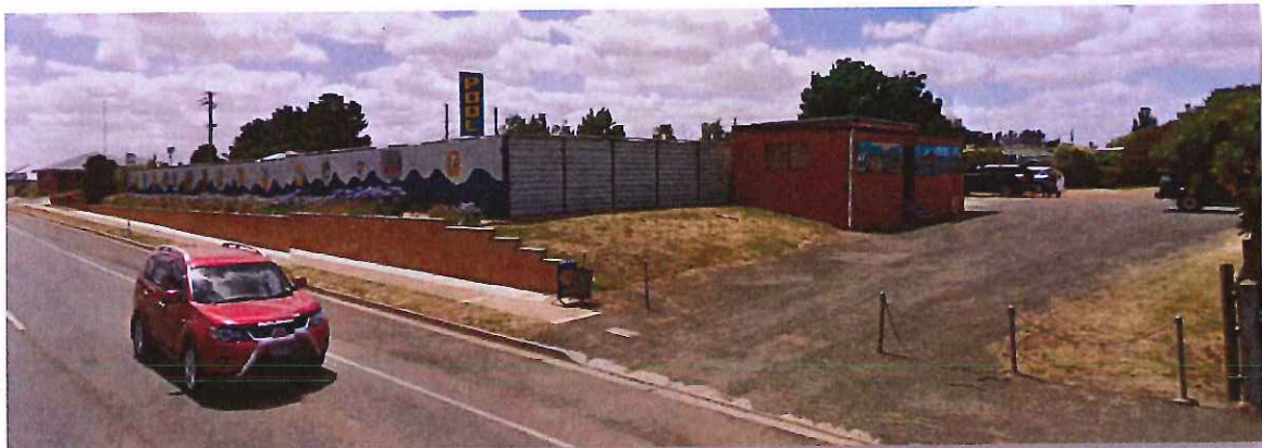
Figure 2 – Existing access and parking from Main Street
