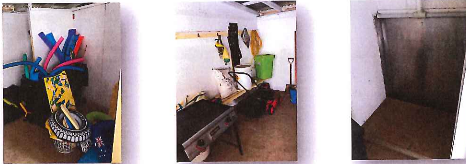
Figure 8 – Existing amenities are outdated and currently used for storage of most maintenance and safety equipment.
