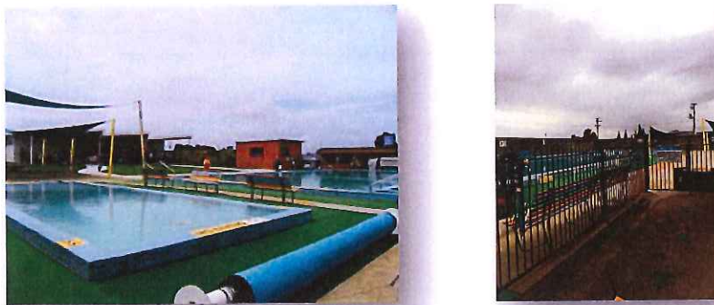
Figure 4 – Pool capping and concourse require upgrading to safer options.
