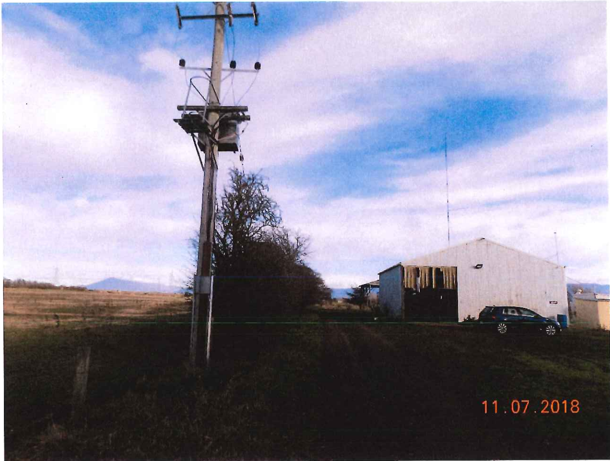
Existing access driveway to site from Green Rises Road
