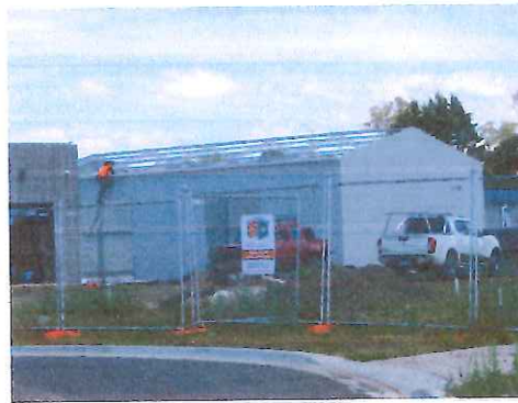
Another much larger shed in the local area
