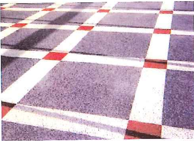
Fig. 6-19. Red and blue pigments were used to color this terrazzo floor. (69873)
