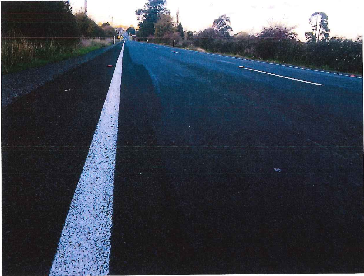
Evandale Main Rd shoulder widening works
