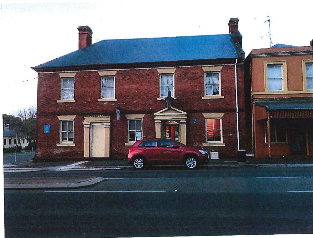
Photograph of subject site
