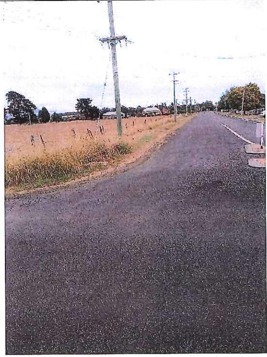
Figure 4 - Looking west along Bulwer Street.
