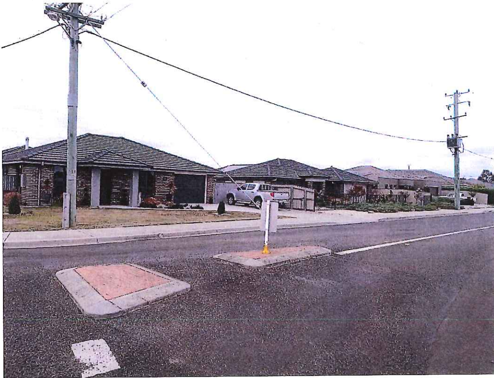
Figure 11 – residential houses on the east of Catherine Street.
