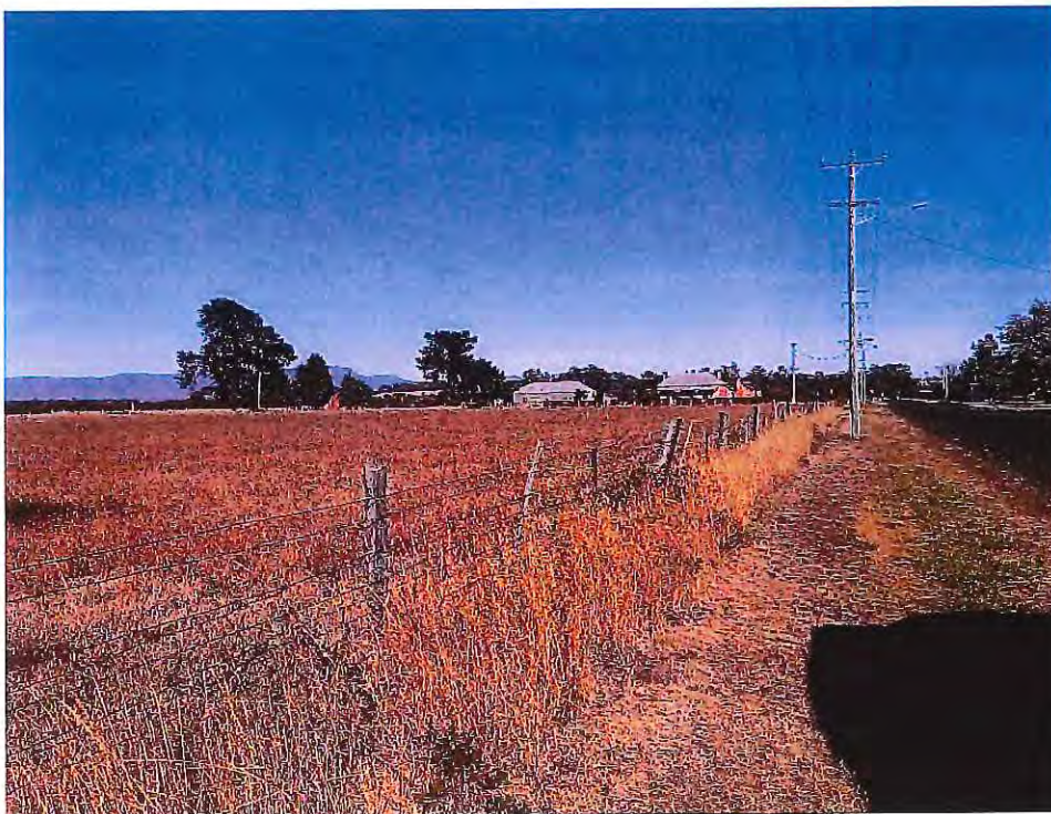
Corner of site and Bulwer St
