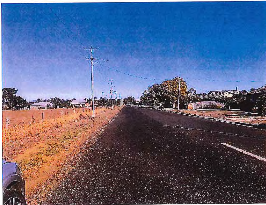
Figure 7 – Bulwer St looking west
