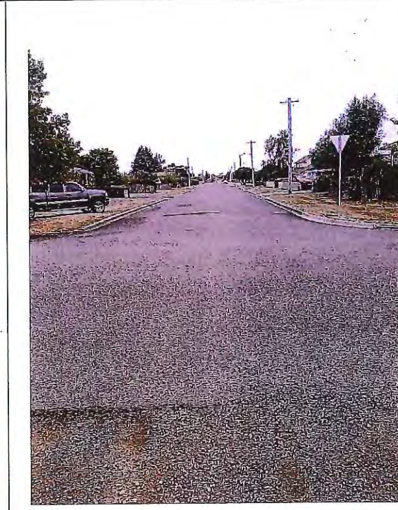
Figure 6 - looking north along Burghley Street
