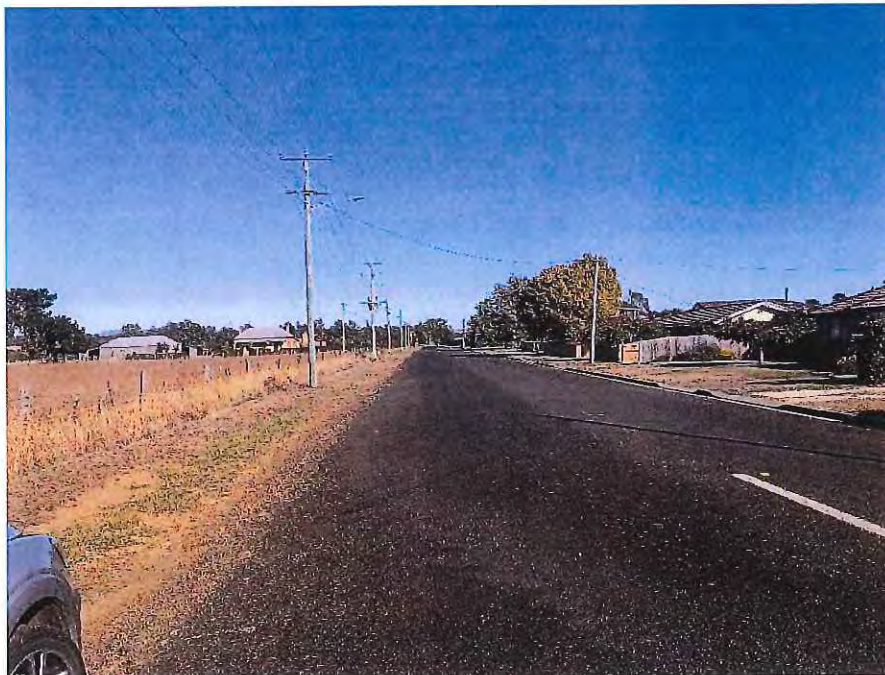
Figure 7 – Bulwer St looking west
