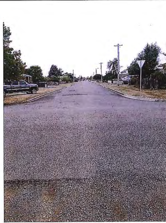
Figure 6 - looking north along Burghley Street
