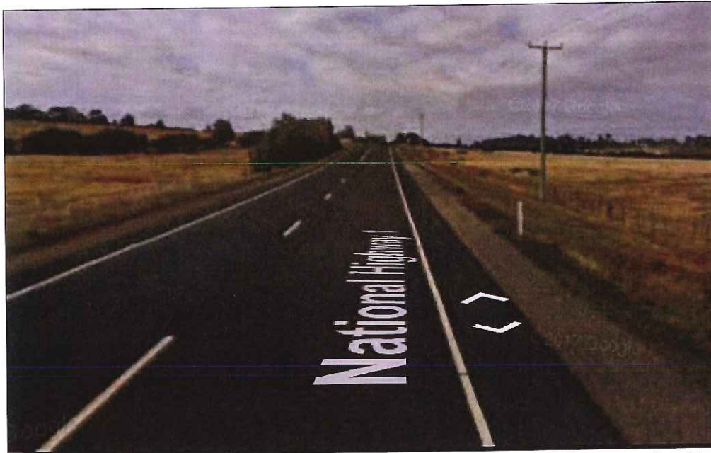
Image 4 – Looking south along the old Midlands Highway. Available sight distance is in excess of 750m from the proposed intersection on the right hand side.
