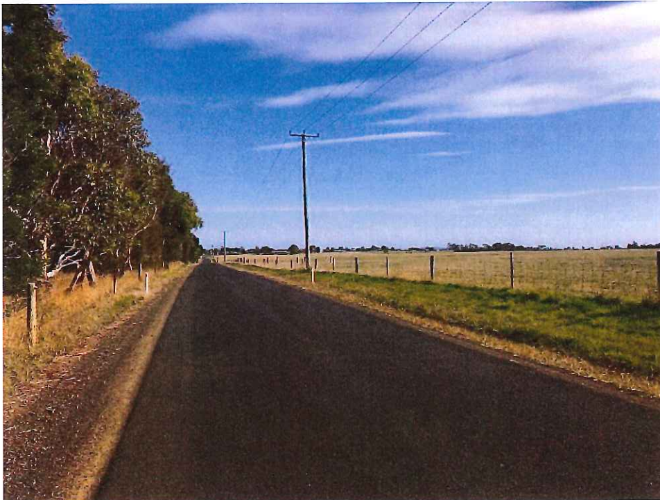
Figure 7: Logan Road - Where Emergency Access to the Site is Proposed
