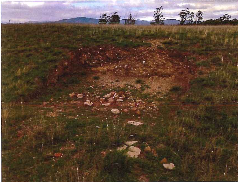
Exposed fill with concrete, brick and glass
