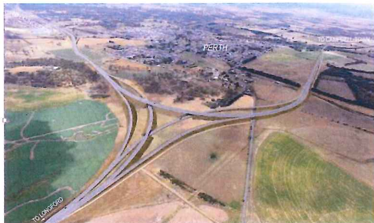
(Source: DSG Midland Highway Safety Upgrades, Perth Link Roads)
