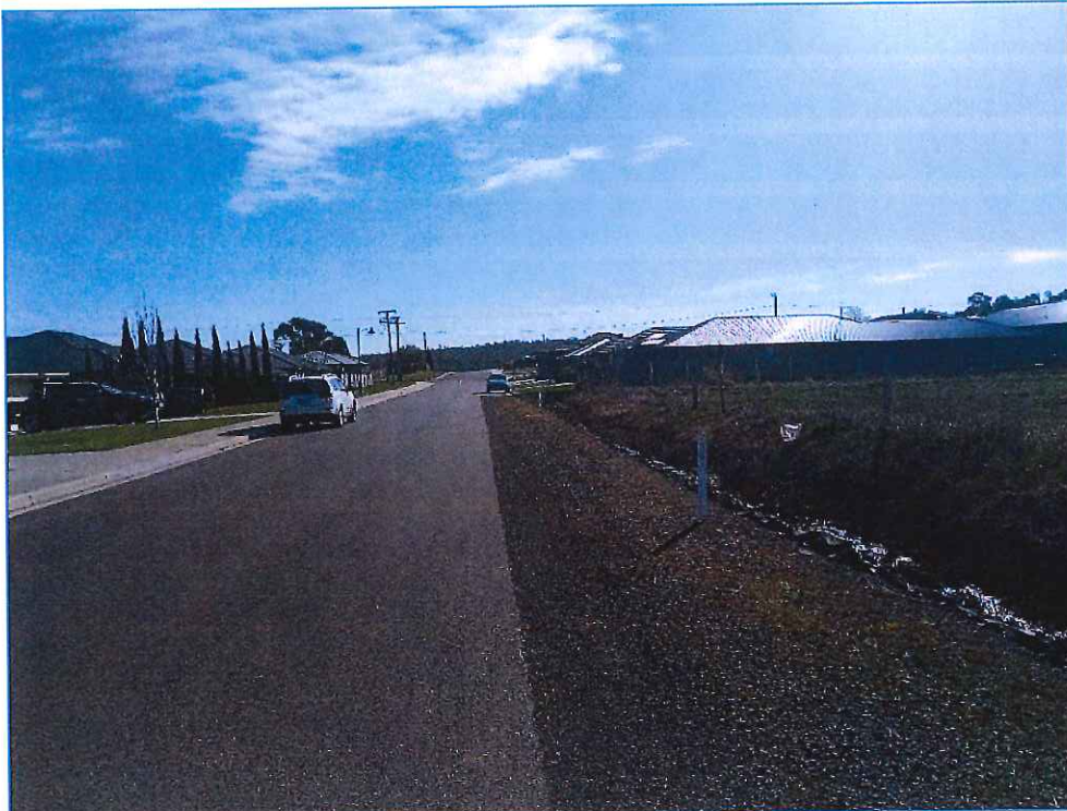
Image 9 – Looking west along Seccombe Street to the Mulgrave Street intersection from the proposed intersection.
