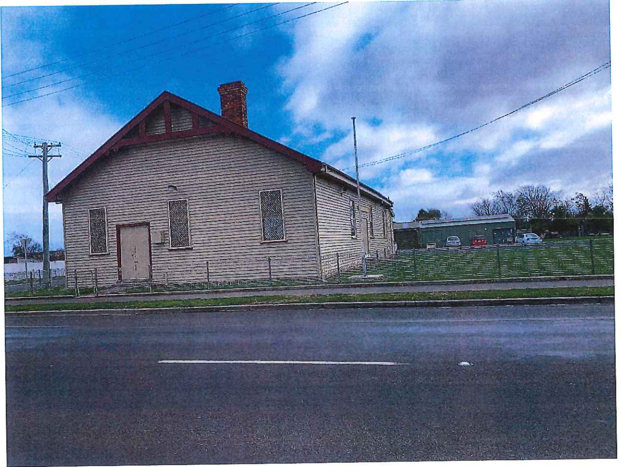
Photo 1: View of site from Marlborough Street
