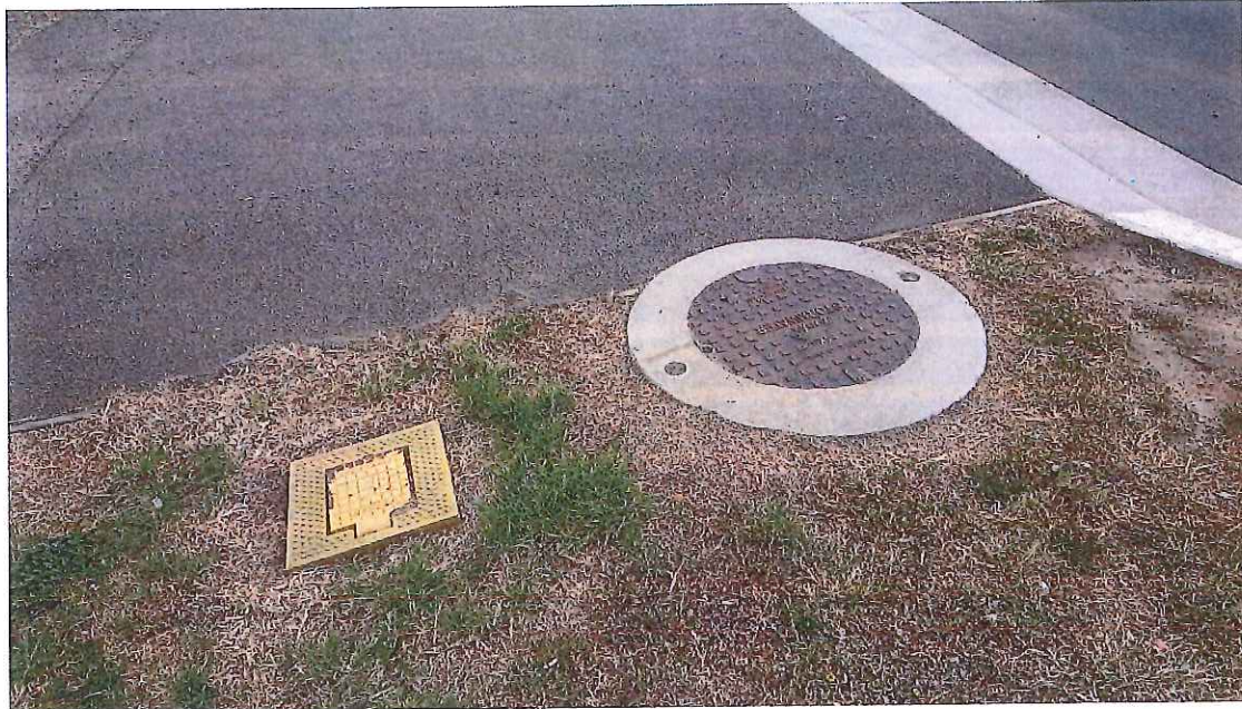
Stormwater manhole north of property
