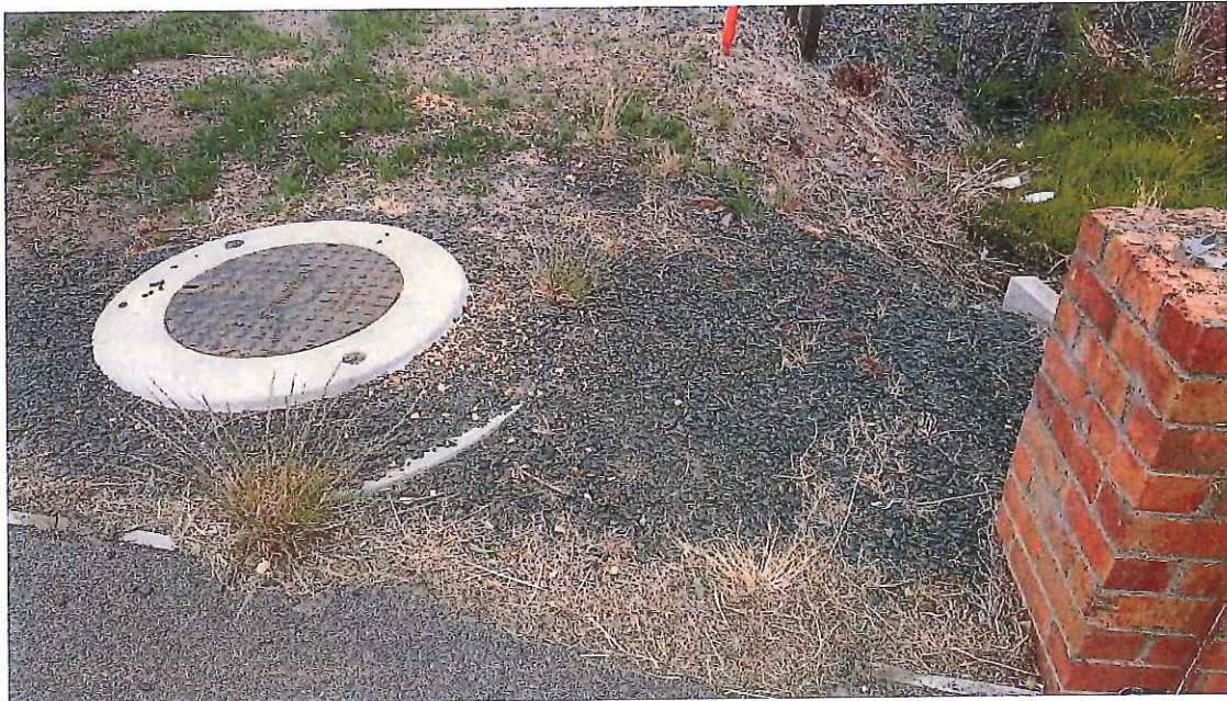
Stormwater manhole east of property boundary
