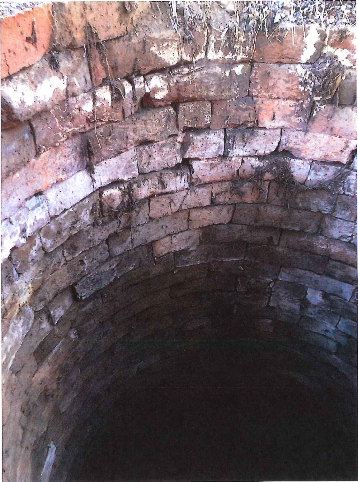
Photo 5 – Close view of well from SW
