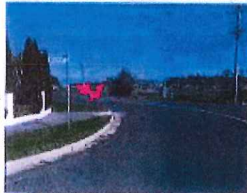
Fig 4.1b - Sight Triangles to Lot 9 access (paved road) from North, considering potential sight distance from nearby intersection with Forest St Road
