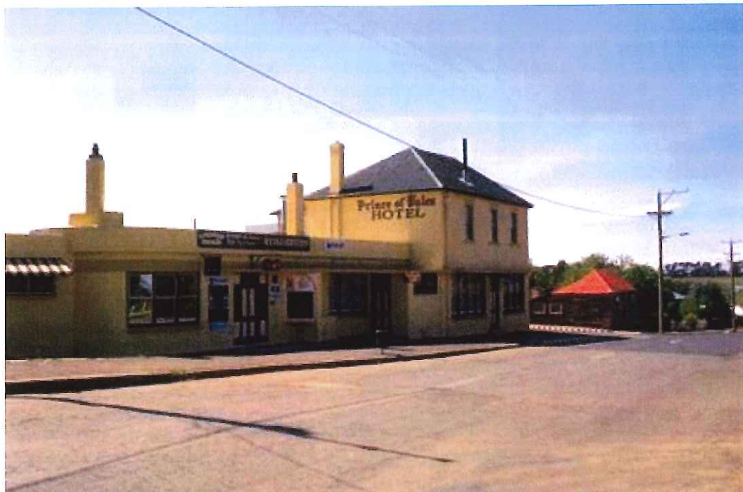
Plate 22: The Prince of Wales Hotel, Evandale
