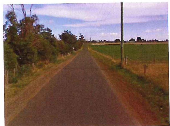
Figure 11: Logan Road - Facing West (Image source: Google Street View, March 2010)
