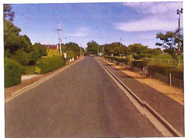
Figure 7: Barclay Street - Facing West (Image source: Google Street View, March 2010)
