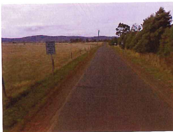
Figure 10: Logan Road - Facing East (Image source: Google Street View, March 2010)
